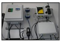
ers can be provided to assist the client in monitoring the quality of both inlet and outlet of the system. Optional instrumentation includes pH, ORP, chlorine, turbidity, and silt density index.
